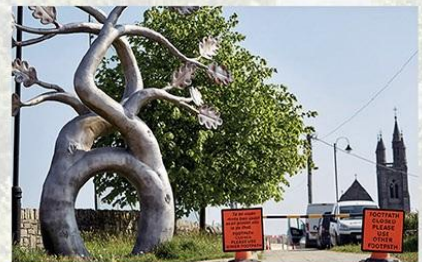
Construction of new footbridge at Ballybofey/Stranorlar Bridge
